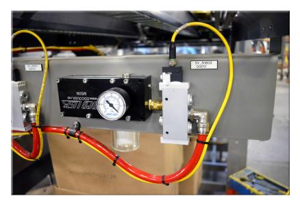
Solenoid valves are electromechanical valves controlled by electrical current through a solenoid coil(s).
