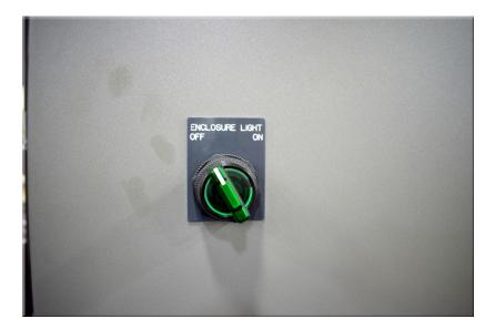
The **Enclosure Light Off/On** selector switches turn the corresponding electrical enclosure's light off and on. The selector switch is illuminated while in the on position.
