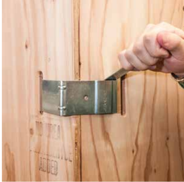
Remove Clips (Start with top clips)
