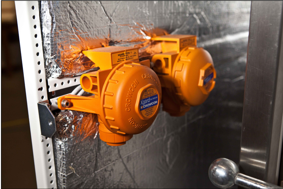
Figure 7:8 Gas detection sensors within Labcat
