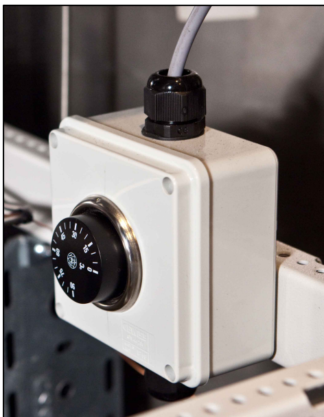
Figure 7:15 Thermostat Control - NOT to be adjusted
