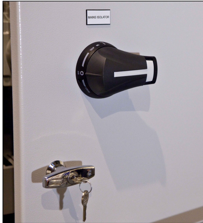
Figure 7:4 Mains Isolator Switch
