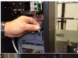
3. PLUG UNIT IN TO EXTERNAL POWER AND TURN UNIT 'ON'. THE INDICATOR LIGHT WILL TURN RED AND SHORT BEEP WILL SOUND.
