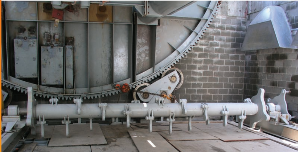
Construction photo of new Hammermill.
