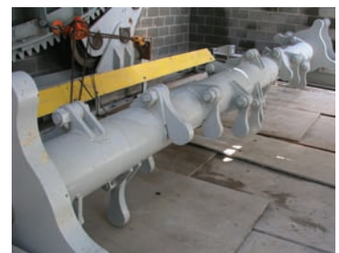
Construction photo of new Hammermill installation.
